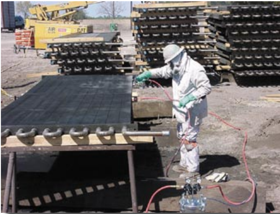
Figure 2. Application of FlueGard-325S on an economiser.
