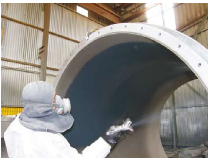
Figure 7. Application on one section of the chimney.
