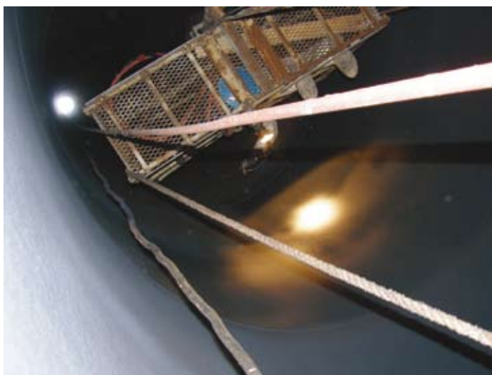
Figure 6. Application in progress.
