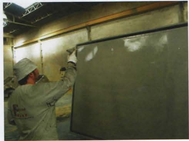
Figure 6. Spray application of CorrosionGard-160S in Spain.
