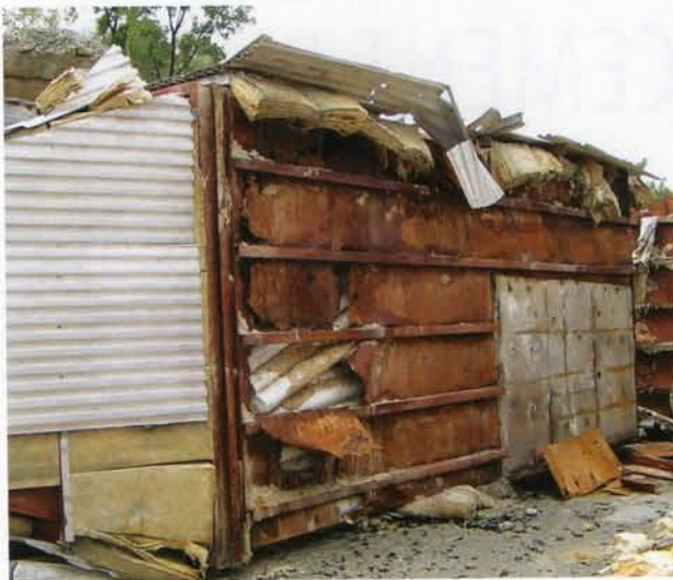
Figure 3. Severely corroded baghouse filter after three years.
