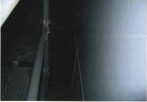
Figure 7. CorrosionGard-160S coating on a waste incineration baghouse in France.
