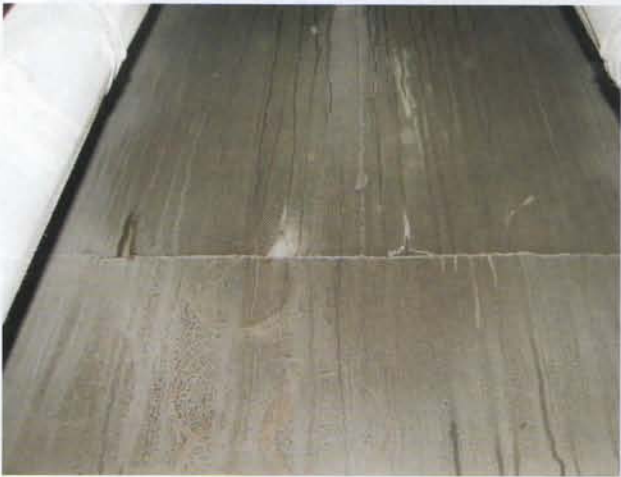
Figure 8. Wall inspection after one year in service, no corrosion.
