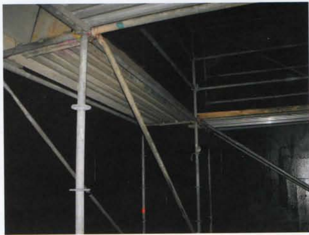
Figure 4. Coating of lower section of a chimney in Missouri.
