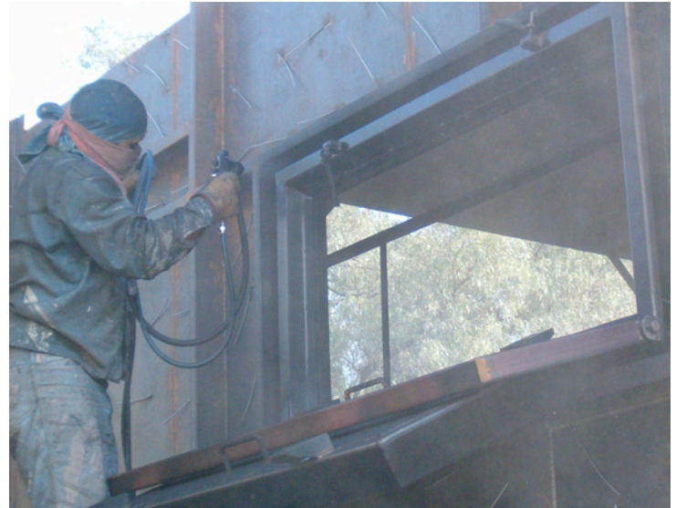
Spray application of CorrosionGard™-50S
