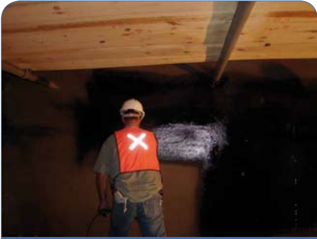
Figure 4. Airless Spray of FlueGard-225SQC in South Africa.
