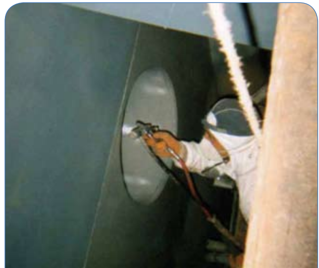
Figure 5. Air spray application of FlueGard-425S in Ireland.
