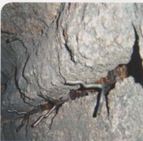
Figure 4. Replacement of damaged anchors.
