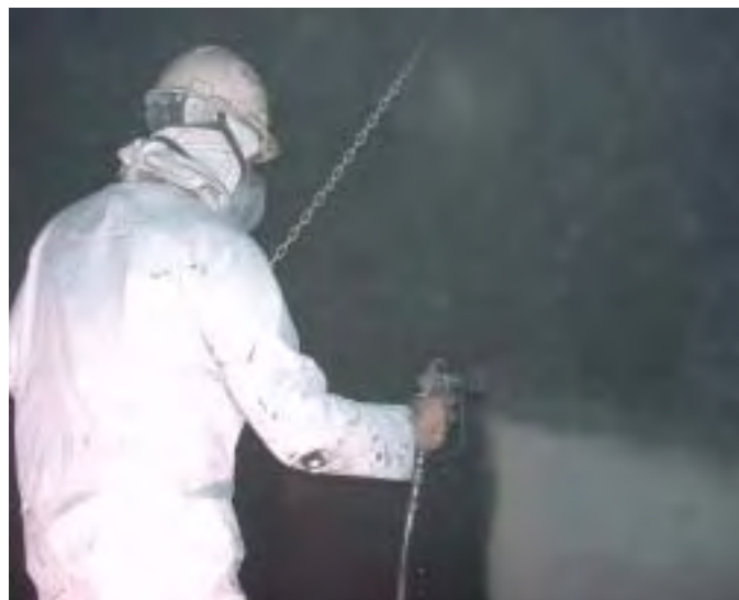
Spray application of FlueGard™-425S
