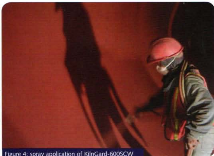
Figure 4: spray application of KilnGard-600SCW
