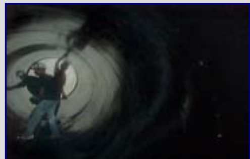
Application of FlueGard™-225S in stack
