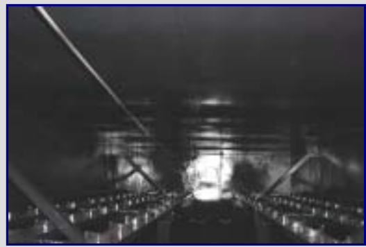
Completed installation of FlueGard™-225S
