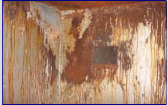
FlueGard™-225S test plate in baghouse
